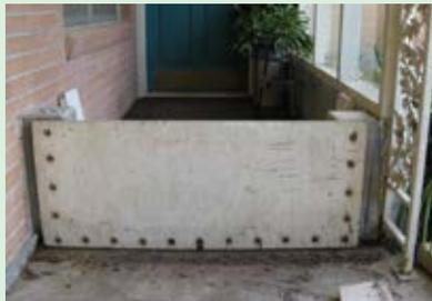
Barriers fabricated to close openings are faster and easier than sandbagging. -French Wetmore
