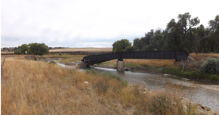
Above: Old Milwaukee Railroad Bridge twisted by flood.
